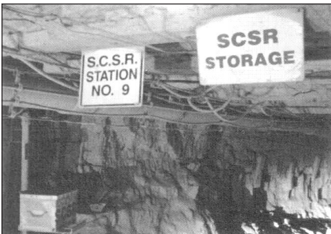
Example of SCSR storage location
